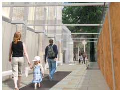
New ambulatory, offices and song school at grade 2 listed St Paul's Knightsbridge.
